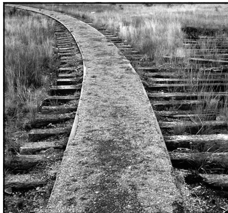
The Kenosha Pass track before the service day. – Photo © Bruce Nall.
